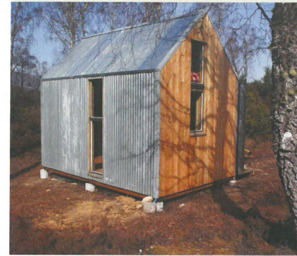
Located within the Cairngorms National Park, Inshriach Bothy was designed by architect Iain MacLeod and artist Bobby Niven. Photo: The Bothy Project.
